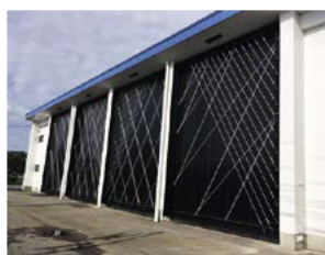
Seismic reinforcement with CFRP rod
